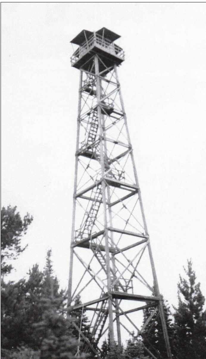
The Black Butte fire watch tower, built by men from the CCC camp, Camp Sisters. JCHS photo
