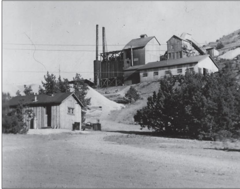
Horse Heaven 'Herreshoff' furnace for smelting mercury on-site
