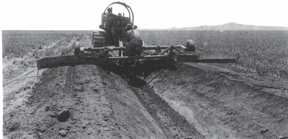
Digging a lateral ditch on Agency Plains, 1948
