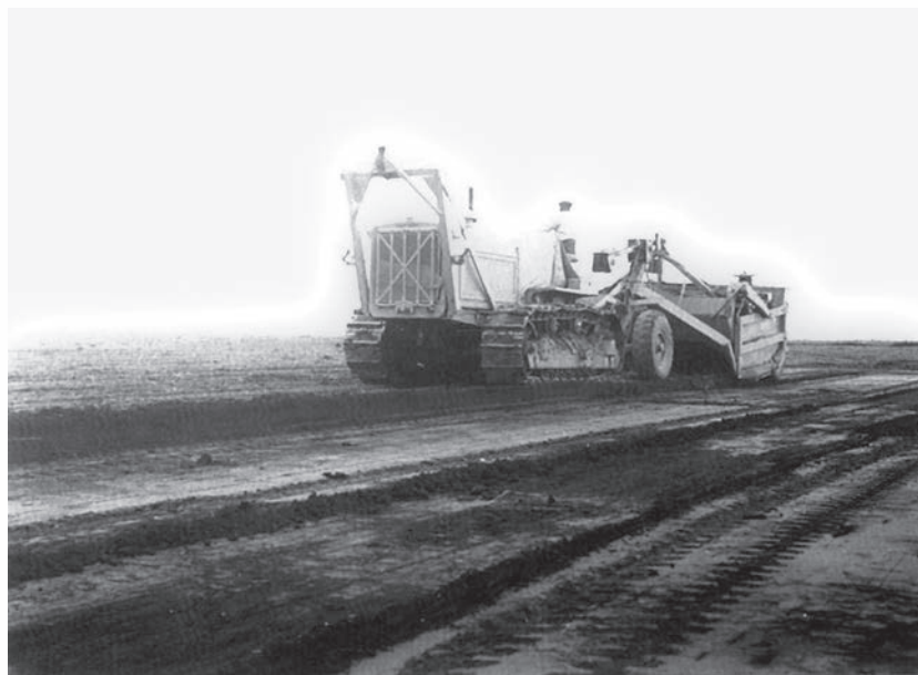
Land-leveling at C.W. Van Cleef farm on Agency Plains (B. of R. photo)
