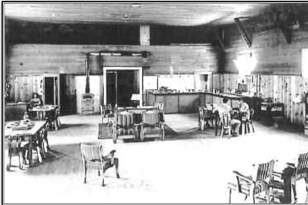
Interior of the Madras USO Center.
